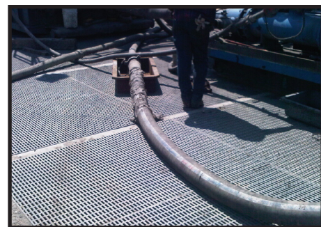
Spill containment system beneath equipment
