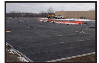
Full Site Containment
