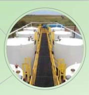
Fibertred<sup>®</sup> stair treads and Fibergrate moulded grating provide corrosionresistant walkways and platforms throughout chemical facilities.
