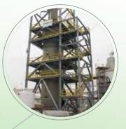
Fiberbrate<sup>®</sup> moulded gratings and stair treads provide access platforms to chemical facility buildings and processing equipment. Dynarail<sup>®</sup> ladders and railings also ensure safety for workers. Fibergrate<sup>®</sup> High Load Capacity moulded and pultuded gratings are used over trenches and can withstand heavy vehicle loads.
